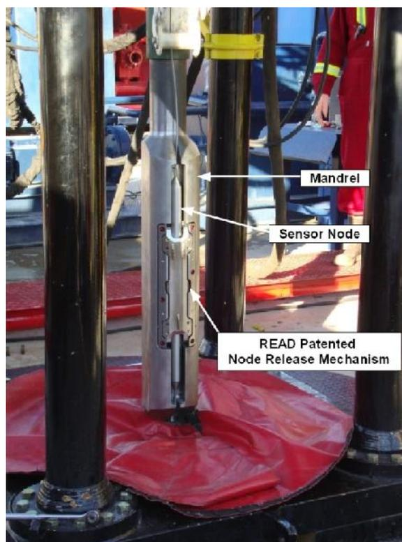
**Figure 5.** *Installing a PerForM™ sensor node on production tubing.*
